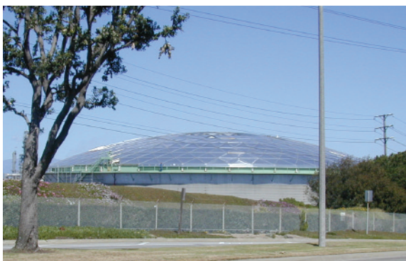
Dome on Tank 1003, located near Rosecrans Boulevard and Bell Avenue.
