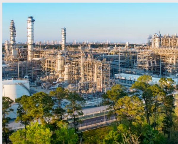
Photo: CPChem successfully applied the MarTECH loop slurry technology in the two polyethylene units as part of the U.S. Gulf Coast Petrochemicals project.
