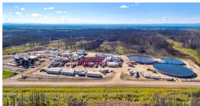
Photo: Horizontal appraisal drilling progressed in the Liard Basin in 2018.
