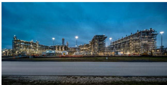
Photo: Start-up of the new ethane cracker was achieved at CPChem's U.S. Gulf Coast Petrochemical Project in March 2018.
